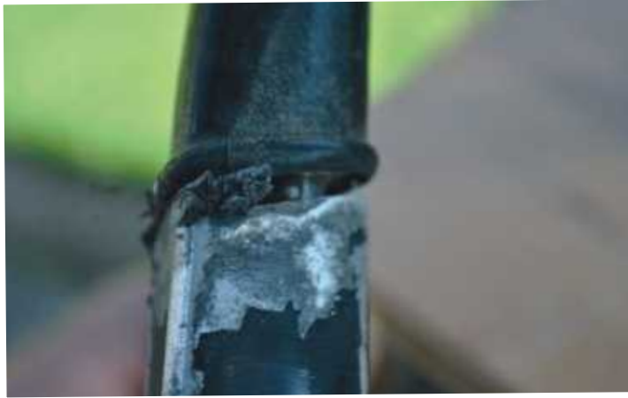
11 Ram the putty to the bottom of the cracks so that it adheres to the steel rod.
