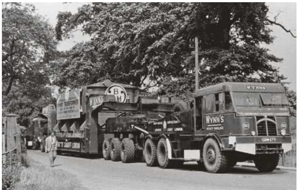
▲ Into the '50s, Wynn's was operating this six-axle Crane girder trailer seen enroute to Staythorpe in Nottinghamshire with a 140 tons transformer.
