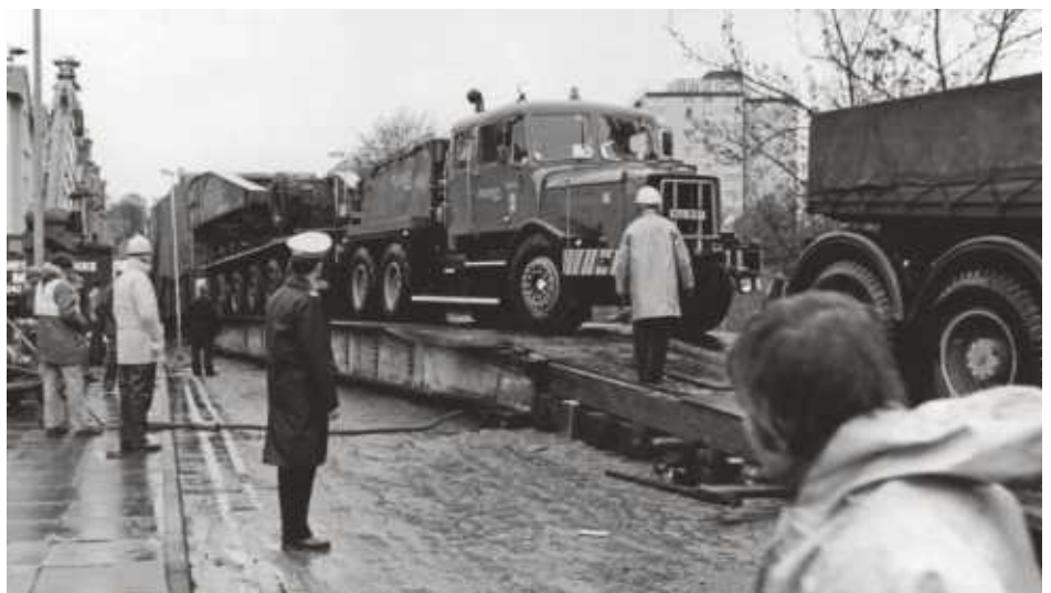
▲ This is a great example of a bridging raft. The roadtrain weight was close to 500 tons and the inner stator core was destined for Inverkip power station. The rather weak railway bridge was on Cardwell Road in Gourock and the bridging raft ensured none of this weight was transferred to the weak bridge.
