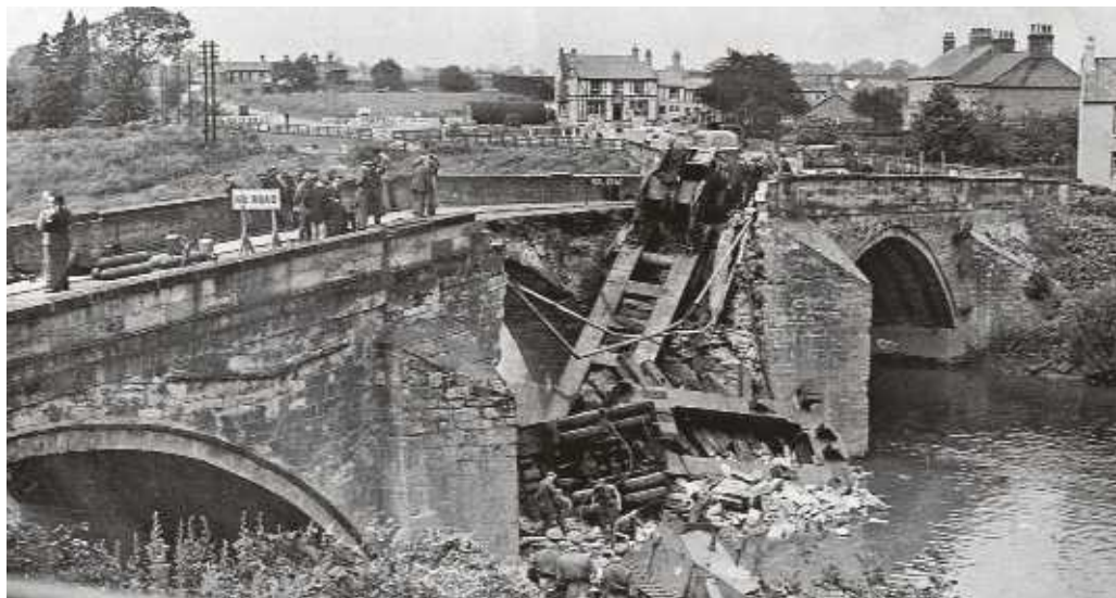
▲ The A1 at Boroughbridge over the River Ure when it collapsed in 1945.
