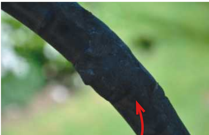
13 Fill the crack so that it is proud of the finished surface.
