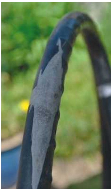
15 Going through the grades as the repair is sanded will give a finish ready for painting in black gloss.
